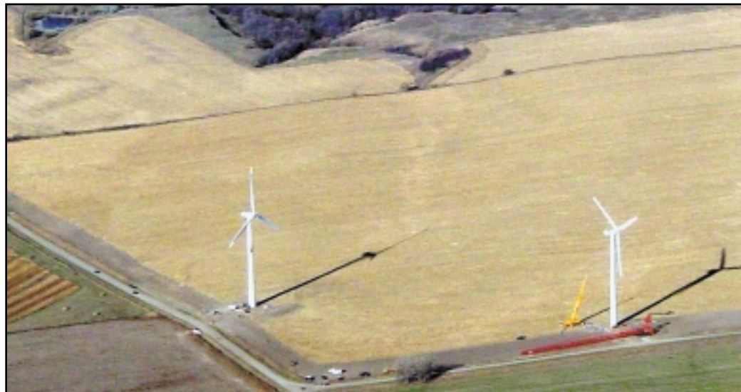
The South Dakota prairie provides an ideal location for these wind turbines, capable of generating a combined 2.6 megawatts. The immense size of the windmills (facing page) is evident from this perspective. When wind speeds become too high, airfoil tips are rotated to act as air brakes. Photos courtesy Basin Electric Power Cooperative.
